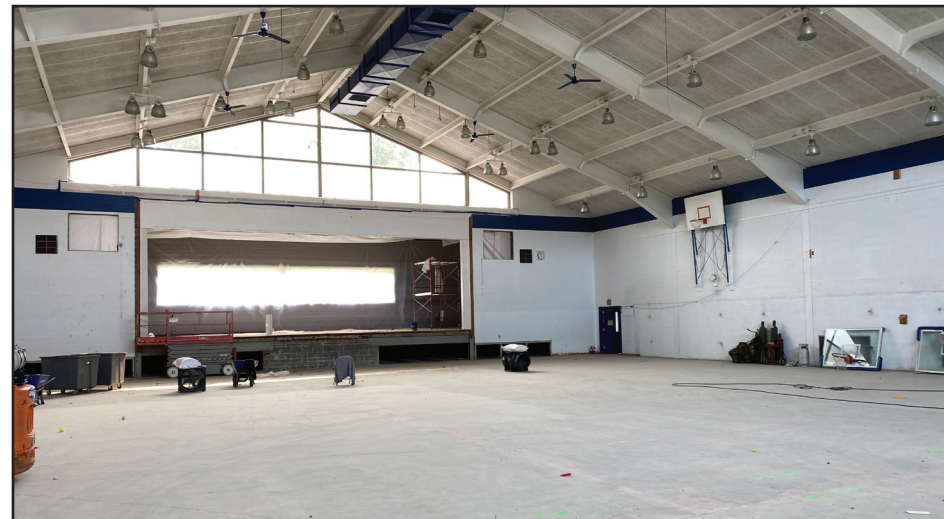
Above: This photo from Sept. 16, 2020 shows what the former gymnasium/auditorium of the former Monsignor McHugh School looked like before renovations began.
