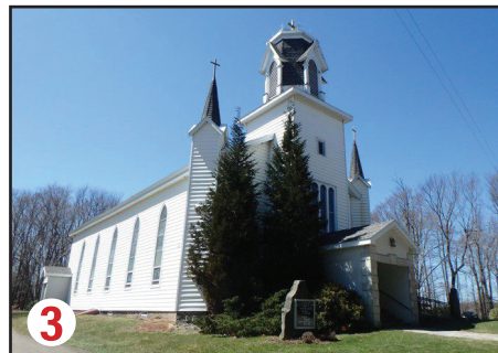
3 Saint Augustine Church 295 Church Road, Brackney
