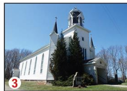
3 Saint Augustine Church 295 Church Road, Brackney
